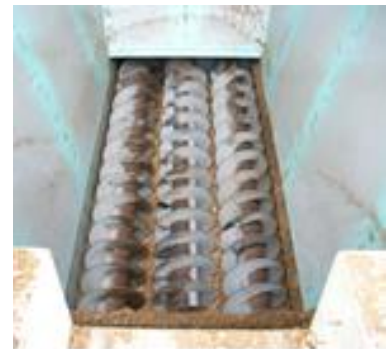
Mounting in discharge screw (wood-fired power plant)
